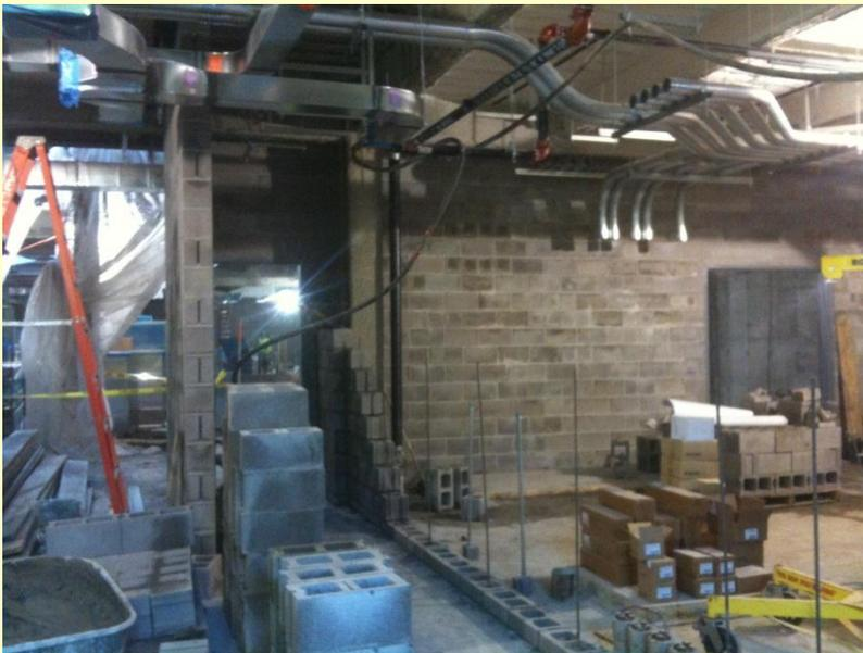
This picture shows how the mechanical systems are underway, with piping for utilities being installed. The cement block wall shown will house the elevator shaft.
